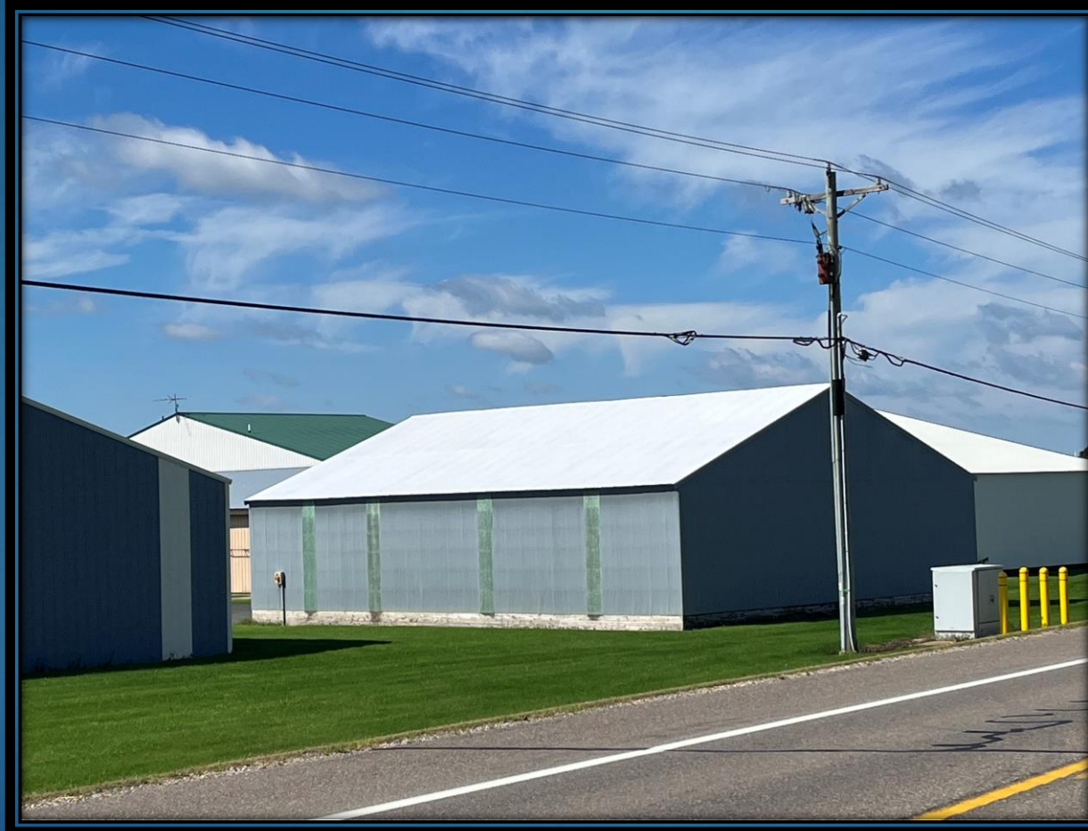
Hangar – New Roof
