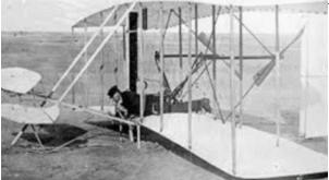
The Wright Flyer I cost about \$1,000 to build (about \$31,500 in today's dollars). The Wright brothers financed the plane entirely by themselves. The framework was made of spruce, with twin "pusher" propellers and a specially designed engine, cast mainly from lightweight aluminum. It was the first controlled and powered flying machine that could fly with the weight of humans. From this design, the modern airplane was born!
