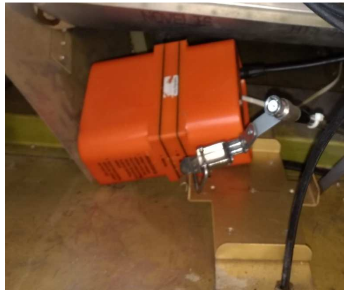
The ELT was rolling around loose in the belly of the plane...
