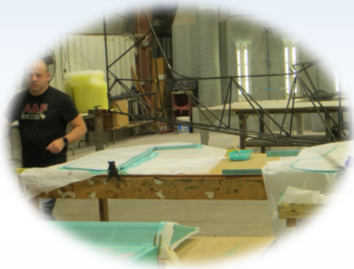
Gluing Covering to control surface
