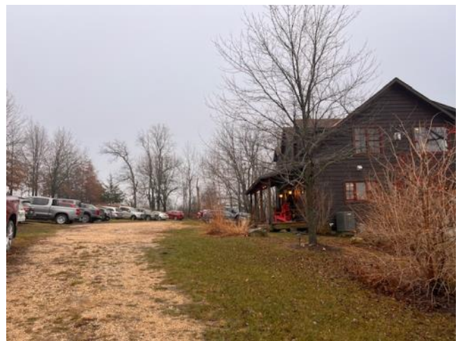
Side view of Rick and Shari Meyer's cabin and parking area
