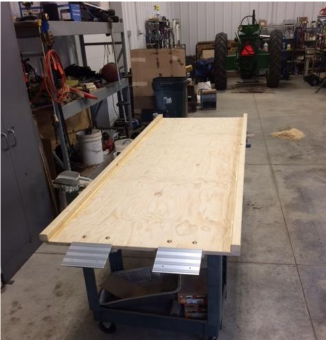
New Ramp for Use at the Repair Barn
