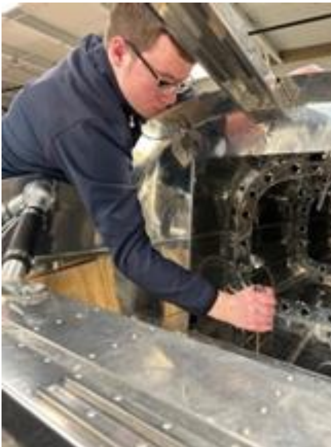
Mathias installing panels.
