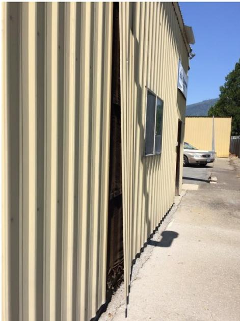
Sometime during the night of July 3 or early the next morning, the wind caught a corner of a sheet of siding on the south wall and pulled it loose. Closer inspection showed some evidence of dry rot, so the attaching screws weren't going into anything solid. Minor repairs have been made to prevent further damage, but a more permanent solution will be required.
