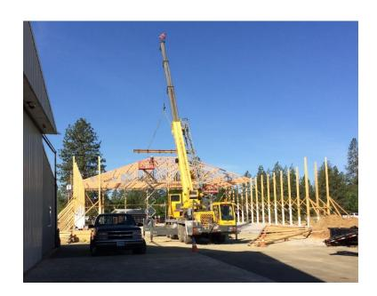
Not every day you see a crane this size on the airport, so I had to get a picture of it while it was there lifting the trusses in place for Sean's new hangar. This structure certainly dominates the skyline as you swing around the south end of the field on Brookside. All the trusses are up now and roofing will soon follow. It should be useable by late July or early August although the interior might not be completely finished by then.
