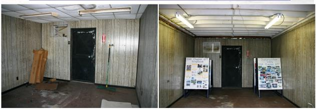
Front room (entrance) water logged ceiling tiles (left) removed, new lights hung (right) and area cleaned up. Being used as temporary storage area for sandwich boards
