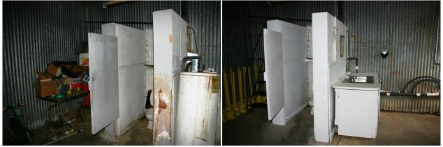
Restroom garbage removed, sink installed, toilet stall repaired and painted.
