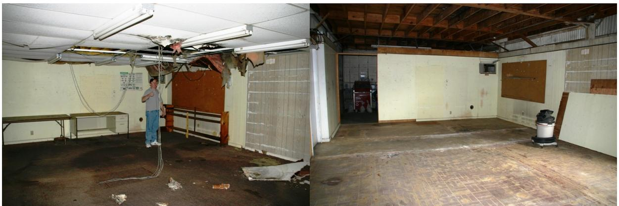
Conference room ceiling, support frame, wiring & carpet removed. Doorway to rest-room and multipurpose rooms cut and framed. Work stopped awaiting roof repair.
