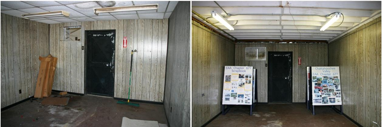
Front room (entrance) water logged ceiling tiles (left) removed, new lights hung (right) and area cleaned up. Being used as temporary storage area for sandwich boards
