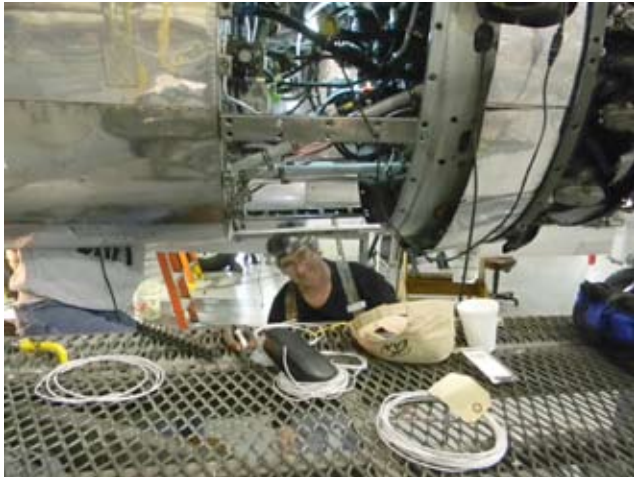
The above picture is Chuck. He and my roommate Bob did the smoke system installation work. Bruce and I, after we finished our job, helped them chase some wires.
