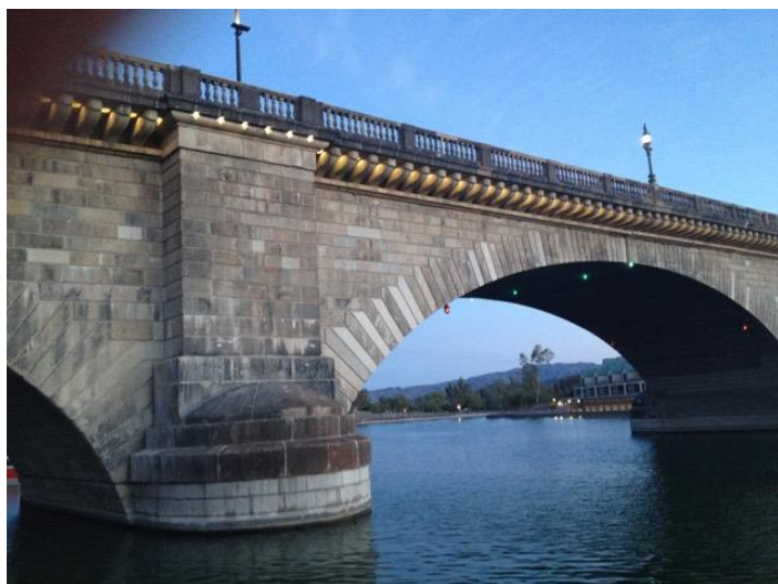
A good shot of the original London Bridge. Dismantled block by block, shipped across the Atlantic Ocean and reassembled in Lake Havasu City.
