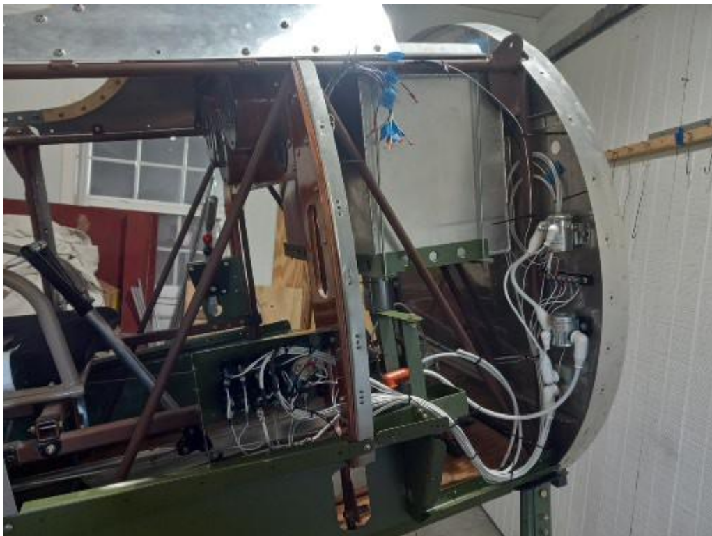
John and his brother Jim have been working on the wiring system.
