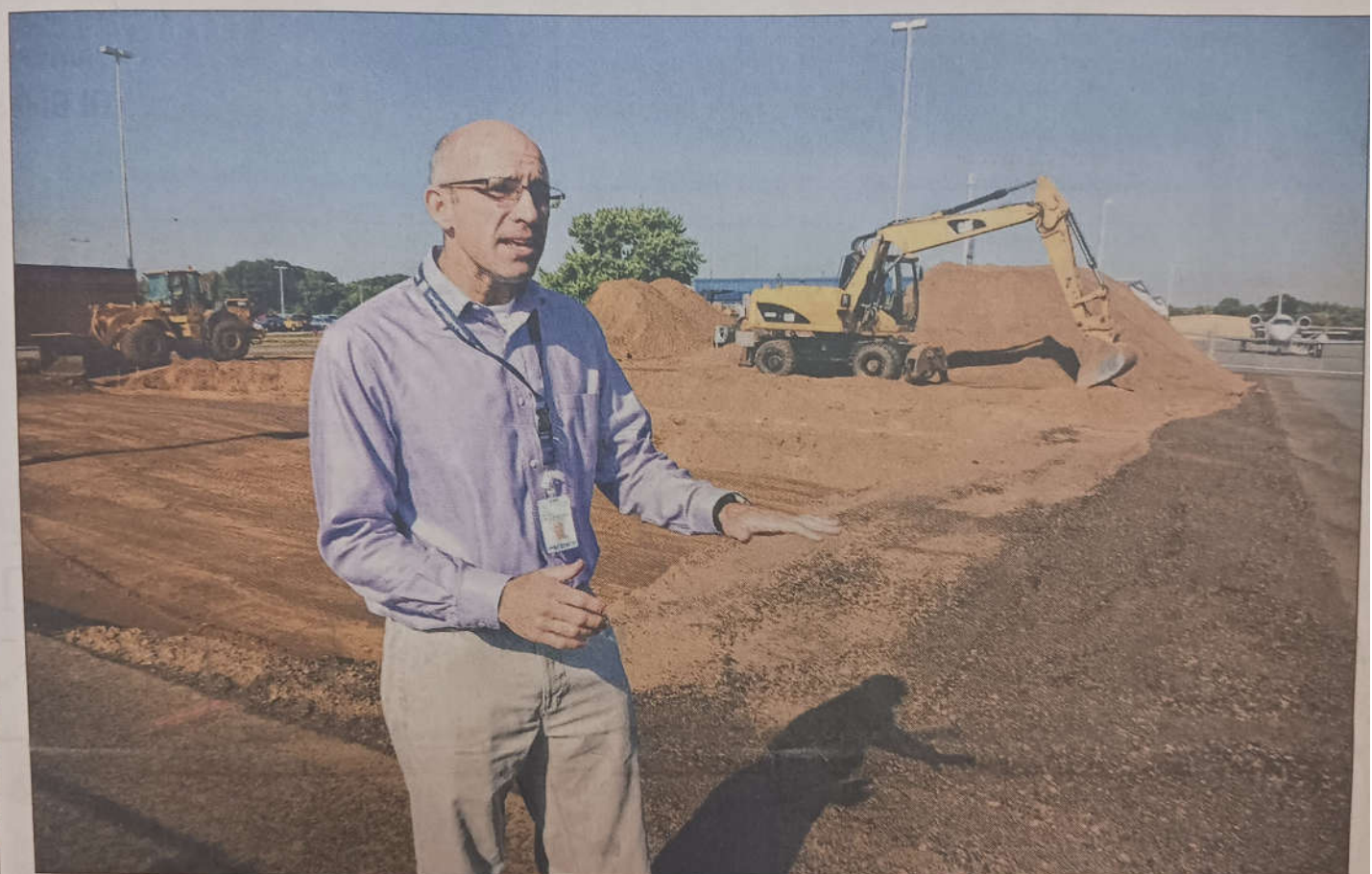
TOP: Private jets wait to be fueled Wednesday at St. Cloud Aviation next to St. Cloud Regional Airport. ABOVE: Bill Towle, director of St. Cloud Regional Airport, talks about projects in the works Wednesday including this hanger under construction. JASON WACHTER, JWACHTER@STCLOUDTIMES.COM
