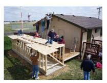
The next phase was attachment of the external sheathing which went fairly quickly. Before the day was done, members hoisted all the roof trusses up on to the building.
