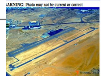
Photo by David Evans Photo taken 27-Apr-2013 looking northwest.
