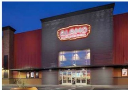
ALAMO DRAFTHOUSE PHOENIX 4955 S. Arizona Avenue Chandler, AZ 85248
