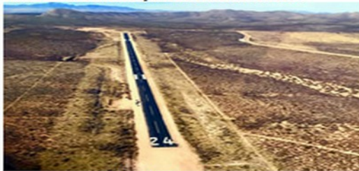
Photo by Trent Thomas Photo taken 02-Mar-2019 looking west.
