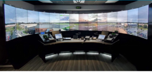
The remote air traffic control system at Leesburg Executive Airport is located in office space along Miller Driver and allows controllers to manage the airspace using video feeds and radar.
