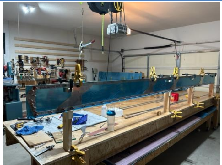
Since I can't move forward with the flaps, I've started on the right main wing spar. Plan to complete both main and rear wing spars before the New Year.
