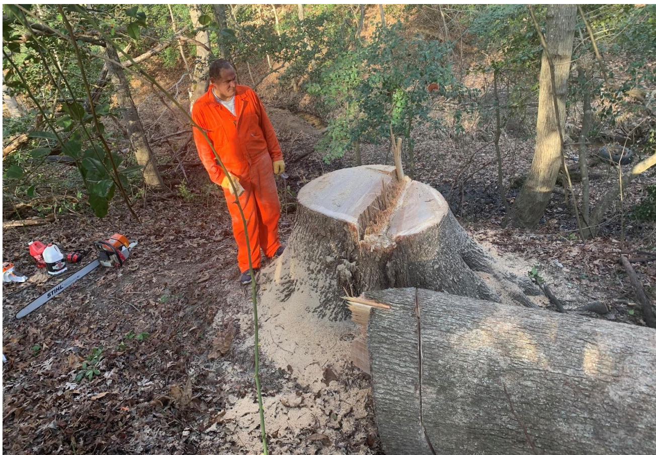
David Rivera working to improve the approaches to the MD50 Runway
