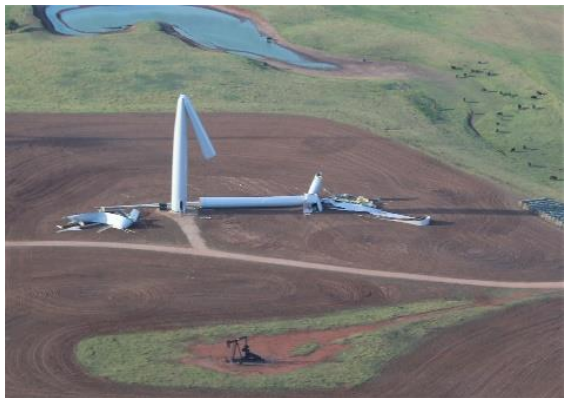
Two recent wind turbine failures near Helena – one tower collapse and one blade failure. The turbine field hasn't been up for very long for these major failures to occur.
