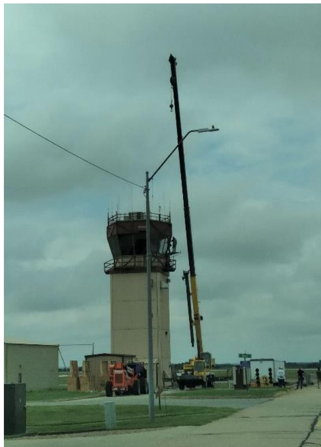
A crane stands along side the tower for lifting the window glass as well as providing an attach point for the installer's safety belt.
