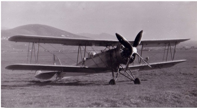
Vet Thomas's Cubby. An experimental amateur built aircraft based on the Piper J-3 Cub
