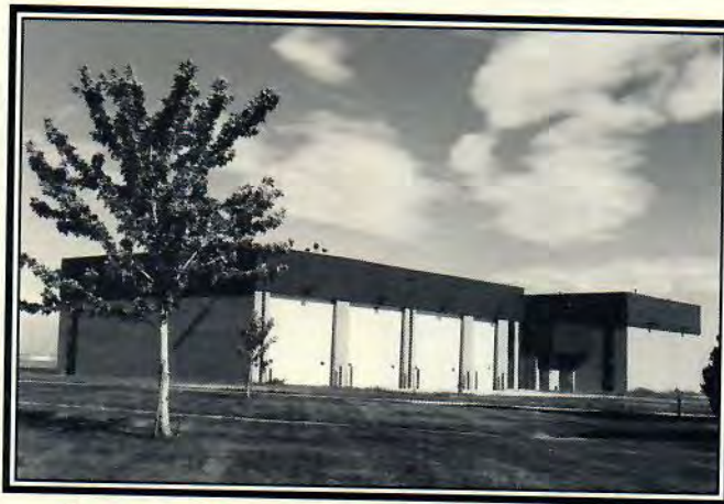
The new maintenance/operations building was completed early this summer.
