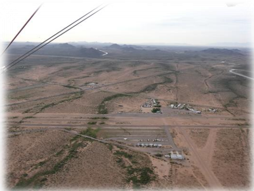
Pleasant Valley Airport north of Phoenix
