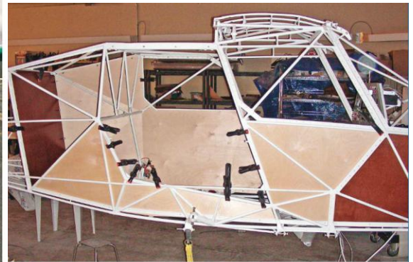
wooden interior being installed inside the steel tube fuselage.
