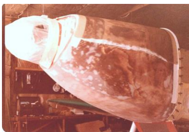
fiberglass layup top half
