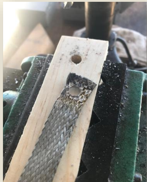
Photo 5: Drilled cable ready to install.
