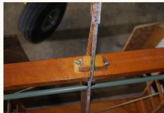
Photo 4: Loose drag wire attachments. Photo credit Doug Jenkins
