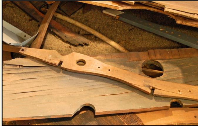
The project has required complete disassembly, cleaning, painting or replacement of each metal piece and nearly every wooden part has had to be re-manufactured. The team has had to carefully research the assembly of the greenhouse, as many parts of the unique element were lost or not original. In a careful reconstruction, every fragment of original wood is valuable as they hold the clues to attach
