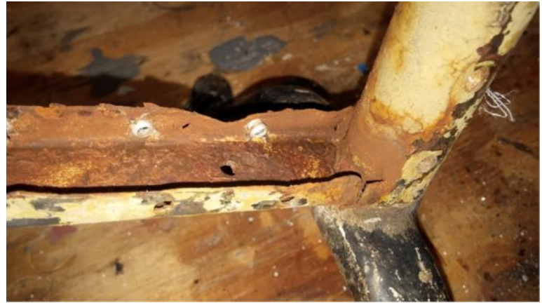
Photo 3: Water trapped at the bottom of this rudder has rusted the structure
