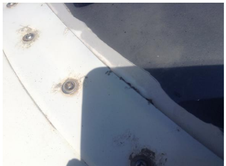
Photo 2: Corrosion around screws attaching a windshield skirt to the fuselage. These screws appear to be from the local hardware store.
