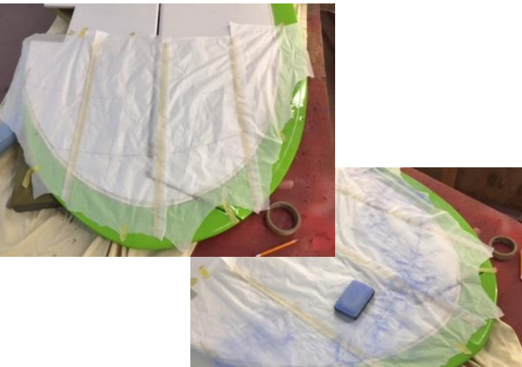
Figures 9, 10, & 11: Perforated tracing paper on the second stabilizer, Pounce pad leaves a dotted line in chalk, tracing paper removed revealing pattern to be masked.
