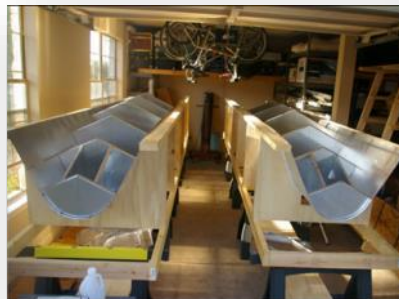
Fabricating and Fitting Bulkheads
