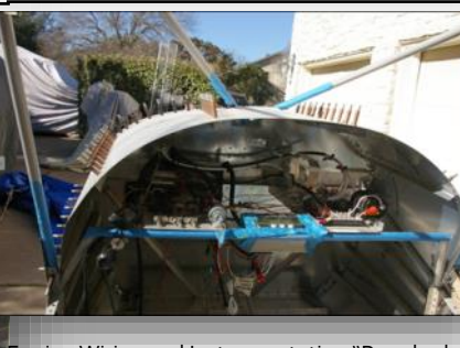
Engine Wiring and Instrumentation "Roughed-In"
