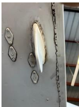
Photo 10: Eroded fairing compound
