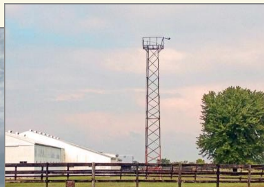
This beacon tower marks a former landing field near Truxton Missouri along I-70.
