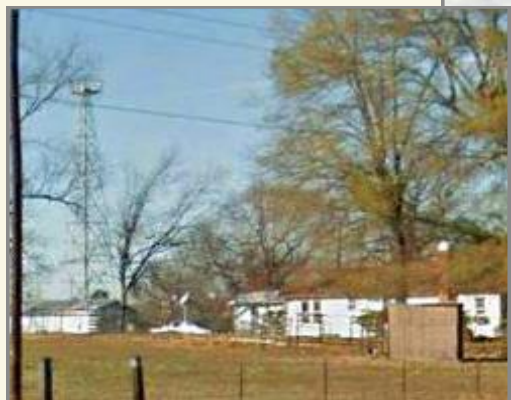
This is a beacon on the Shreveport to Dallas route (along SR 259 north of Judson). One internet contributor says the owner/maintainer has continued to keep this beacon lit. (Image from Google Earth)
