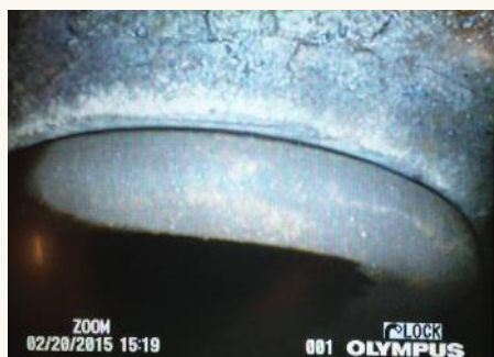
Photo 4: Bore scope look at an exhaust valve (at bottom of frame) resting on the valve seat (at top of frame). The bright white coloration is caused by localized hot gas erosion. Exhaust is escaping past this edge of the exhaust valve. The edge of the valve is rounded and no longer has the squared edge of a good valve.
