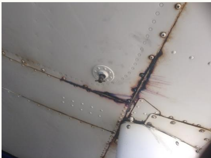
Photo 1: A running fuel leak inside the wing that is seeping out along the sheet metal parting line.
