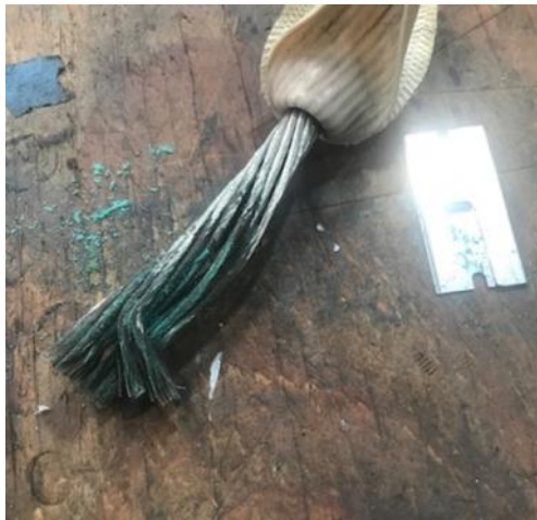
Photo 1: Large diameter corroded wire
