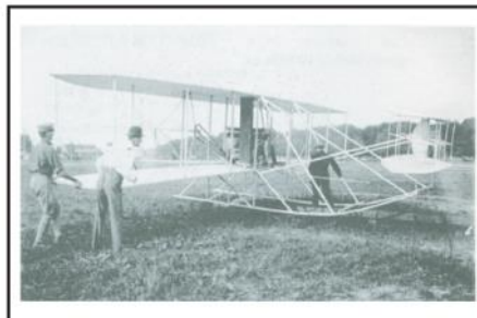
Ground crew placing the plane on the rail
