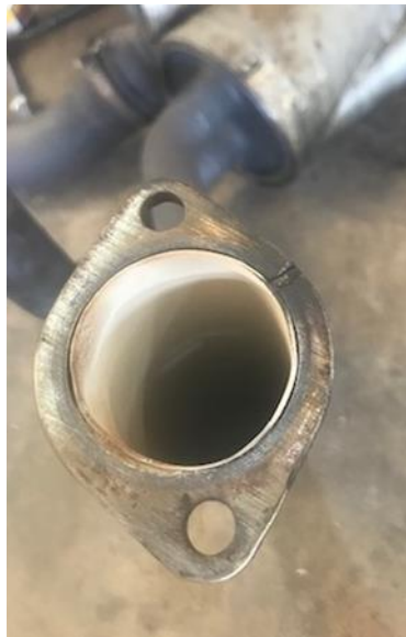
Photo 2: Cracked exhaust flange, and there was an associated distortion in the exhaust gasket.
