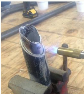
I heat the end of the aluminum. I use Mapp Gas, but use caution because Mapp Gas is quite capable of melting aluminum.
