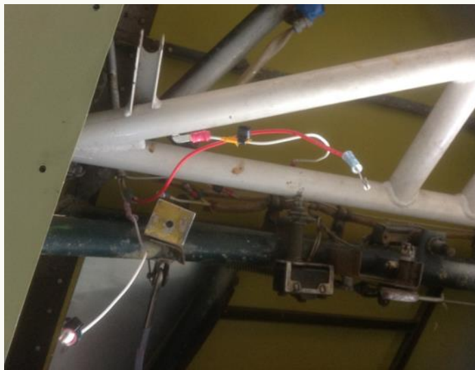
Wires getting connectors. Gear position switches show at
