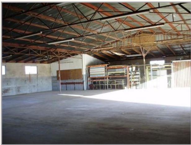
New Digs at Bulverde - Refurbishment in Progress.
