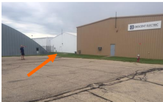
Merle shows Hanger 88 from the road side.
