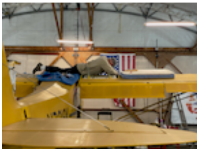
Mark reinstalling fuel tanks
