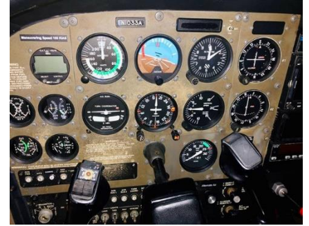
The use of incorrect disinfectant sprayed on an instrument panel damaged a Cessna 172 in the Atlas Aviation fleet at Peter O. Knight Airport in Tampa, Florida. Photo courtesy of Deric Dymerski.
