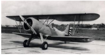
The Waco XPT-14, s/n 39-702, was only slightly altered from standard UPF-7 for Army trainer competition. Narrow tread landing gear was principal recognition feature along with out-of-proportion national insignia.
