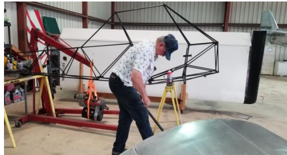
Rheuben Gammel working on the other strut. Work, work, work!
