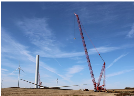
Wind Turbine Farm being constructed N of Beaver Creek, MN
