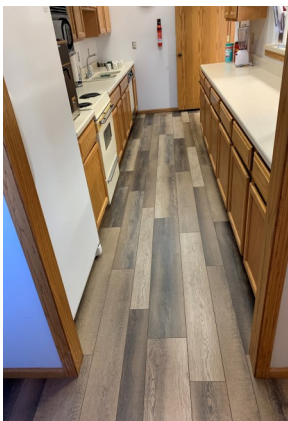
New flooring in Hangar Kitchen
