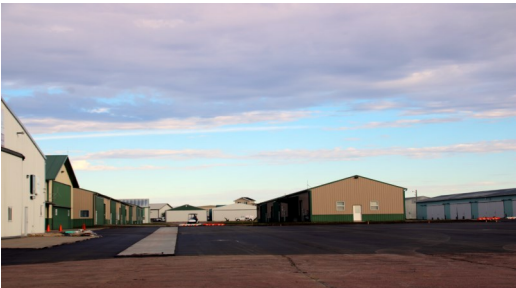
New Parking Ramp at Y-14 October 21, 2023
